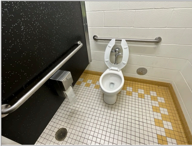
TOILET STALL OVERVIEW
